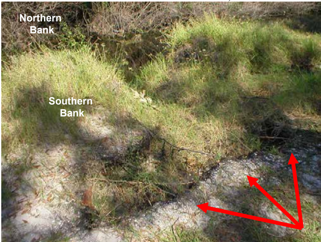
Photo 34 – System 6 - Segment 1 Washout of Southern Bank from Wetland to South, November 2005
