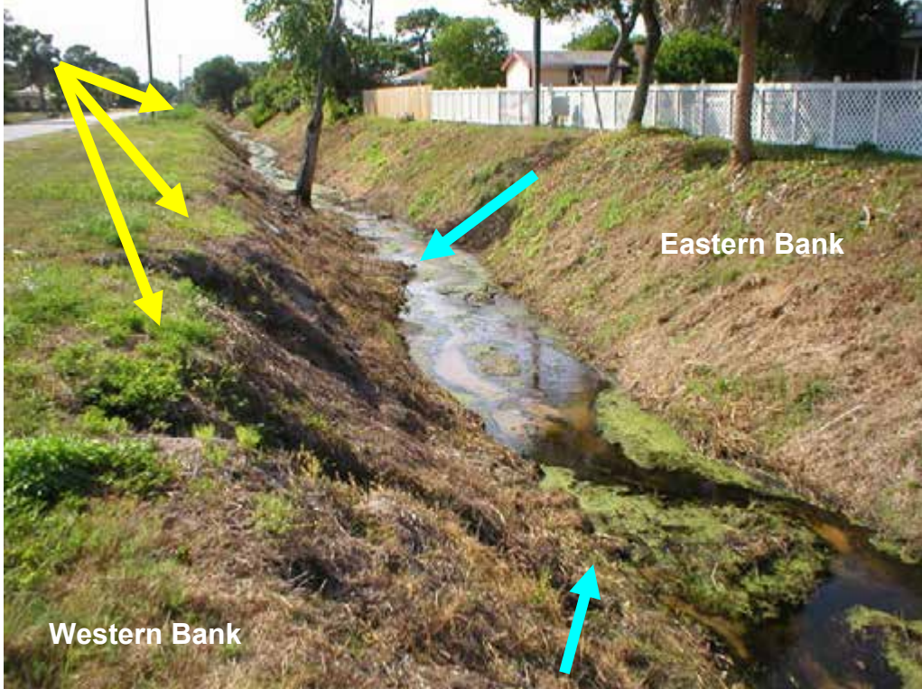
Photo 21 - System 5 - Segment 2 Sloughing Slopes and Sediment Deposition along Western Bank, May 2005
