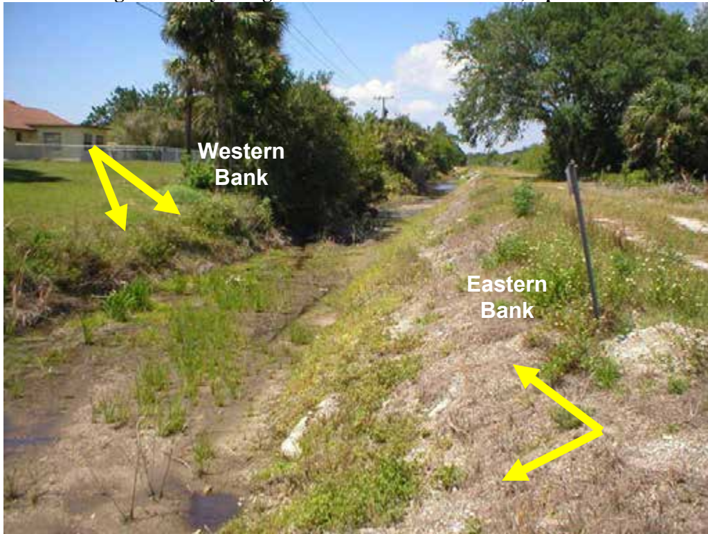
Photo 16 - System 4 – Unevaluated Reach East of Segment 2 Highly Eroded Banks with Variable Vegetative Cover, April 2005
