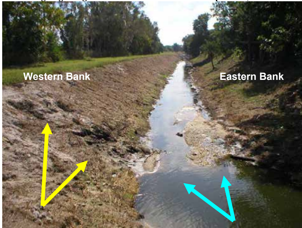
Photo 2 - System 1 - Segment 1 Sloughing along Eastern Bank and Dense Vegetation, May 2005
