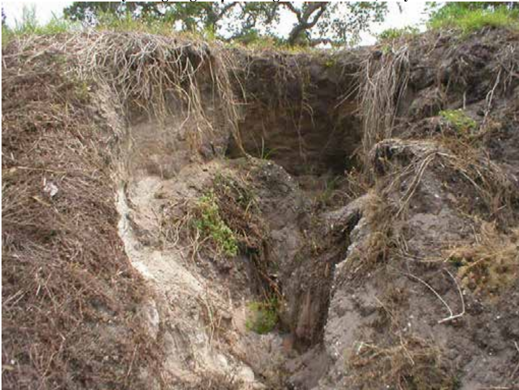
Photo 22 – System 5 - Segment 2 Severely Sloughing Slopes along Western Bank, May 2005
