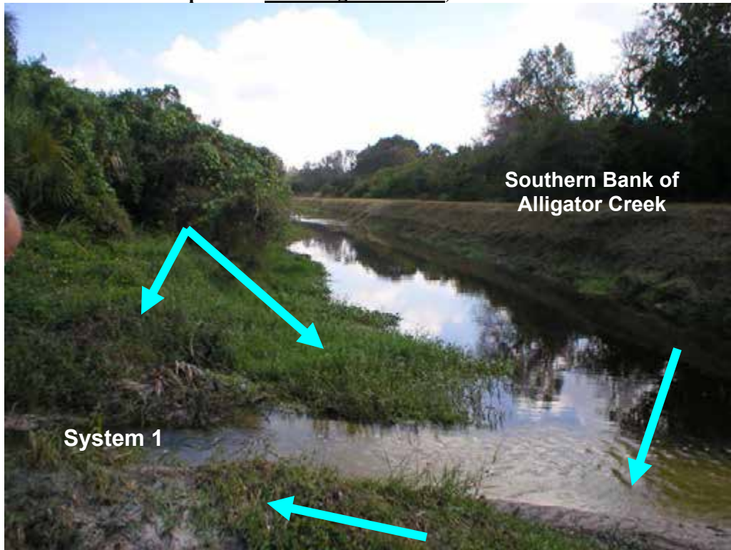
Photo 4 - System 1 - Segment 1 Undercutting of Southern Bank at Alligator Creek, November 2005
