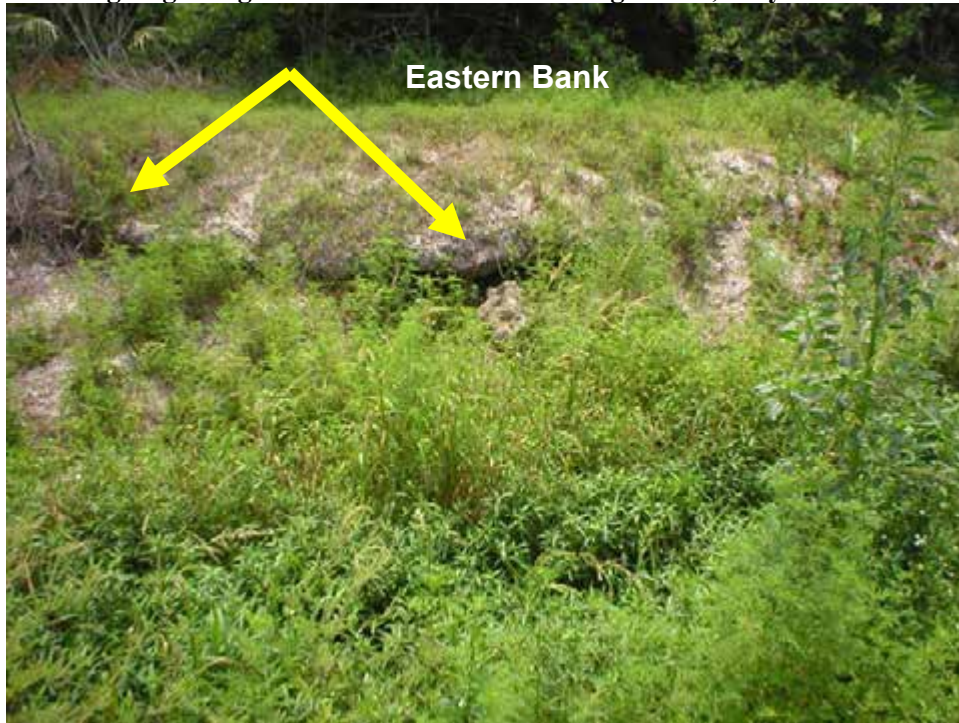
Photo 2 - System 1 - Segment 1 Sloughing along Eastern Bank and Dense Vegetation, May 2005
