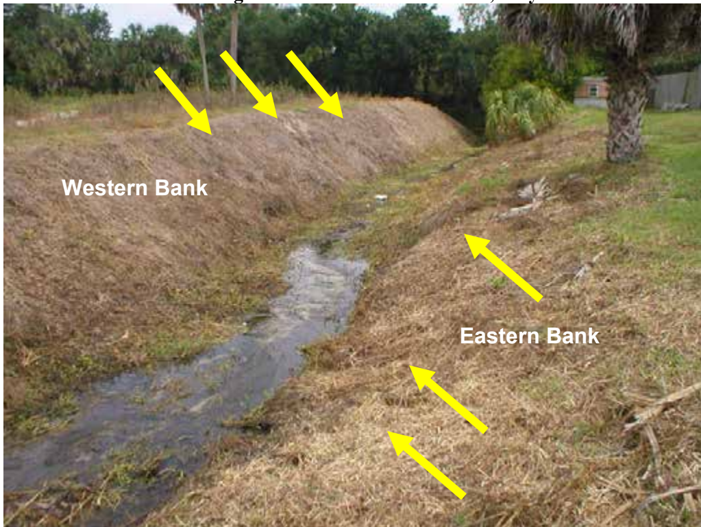
Photo 12 - System 3 Erosion along Eastern and Western Banks, May 2005
