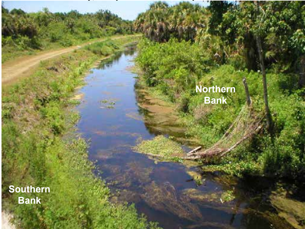
Photo 26 - System 6 - Segment 3 Undercutting of Northern Bank and Sediment Deposition from System 3, July 2005
