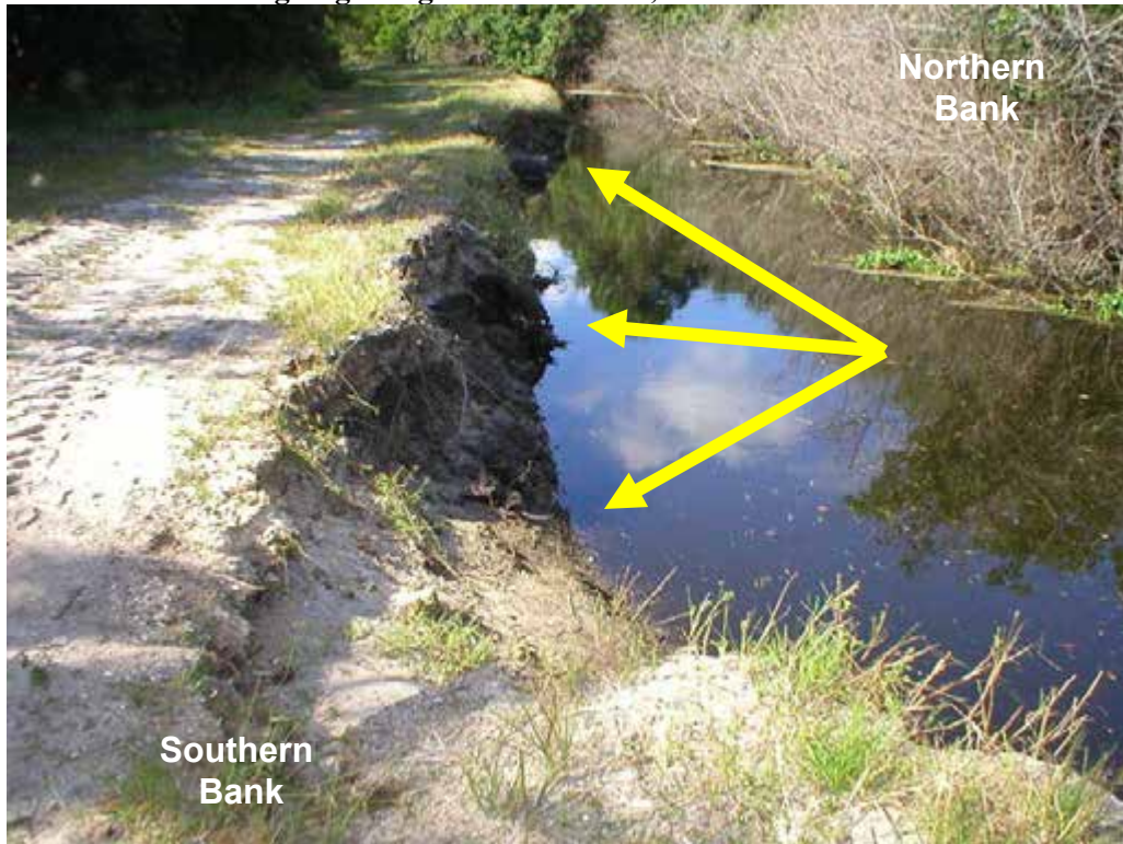
Photo 34 – System 6 - Segment 1 Washout of Southern Bank from Wetland to South, November 2005
