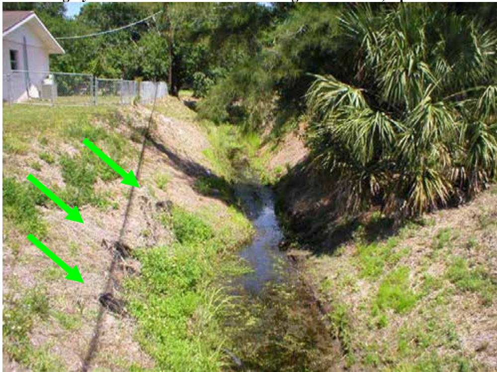
Photo 16 - System 4 – Unevaluated Reach East of Segment 2 Highly Eroded Banks with Variable Vegetative Cover, April 2005
