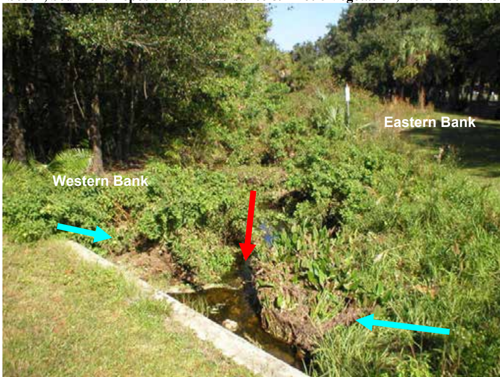
Photo 8 - System 2 - Segment 2 Scour, Sediment Deposition, and Nuisance & Exotic Vegetation, November 2005
