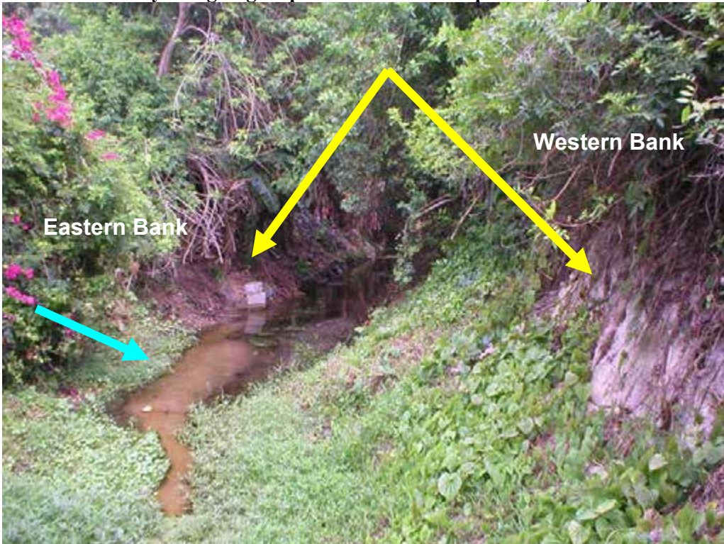
Photo 24 – System 5 - Segment 1 Severely Sloughing Slopes and Sediment Deposition, May 2005
