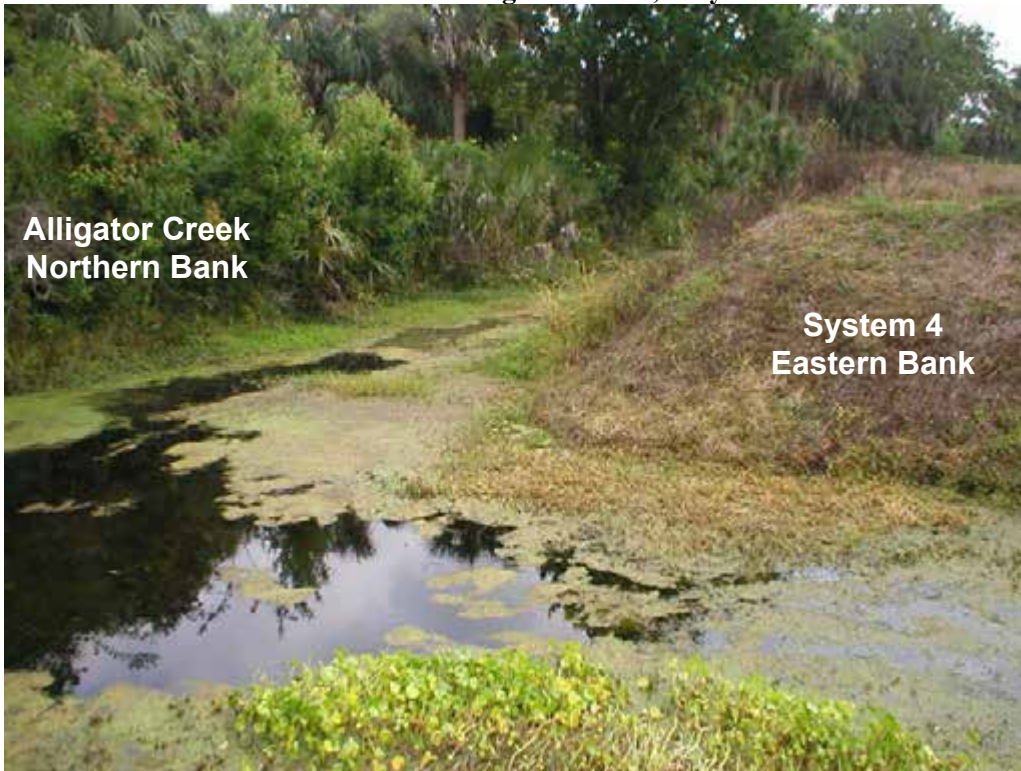
Photo 20 – System 4 - Segment 1 Sediment Deposition (Vegetated) Intersection with Alligator Creek, May 2005
