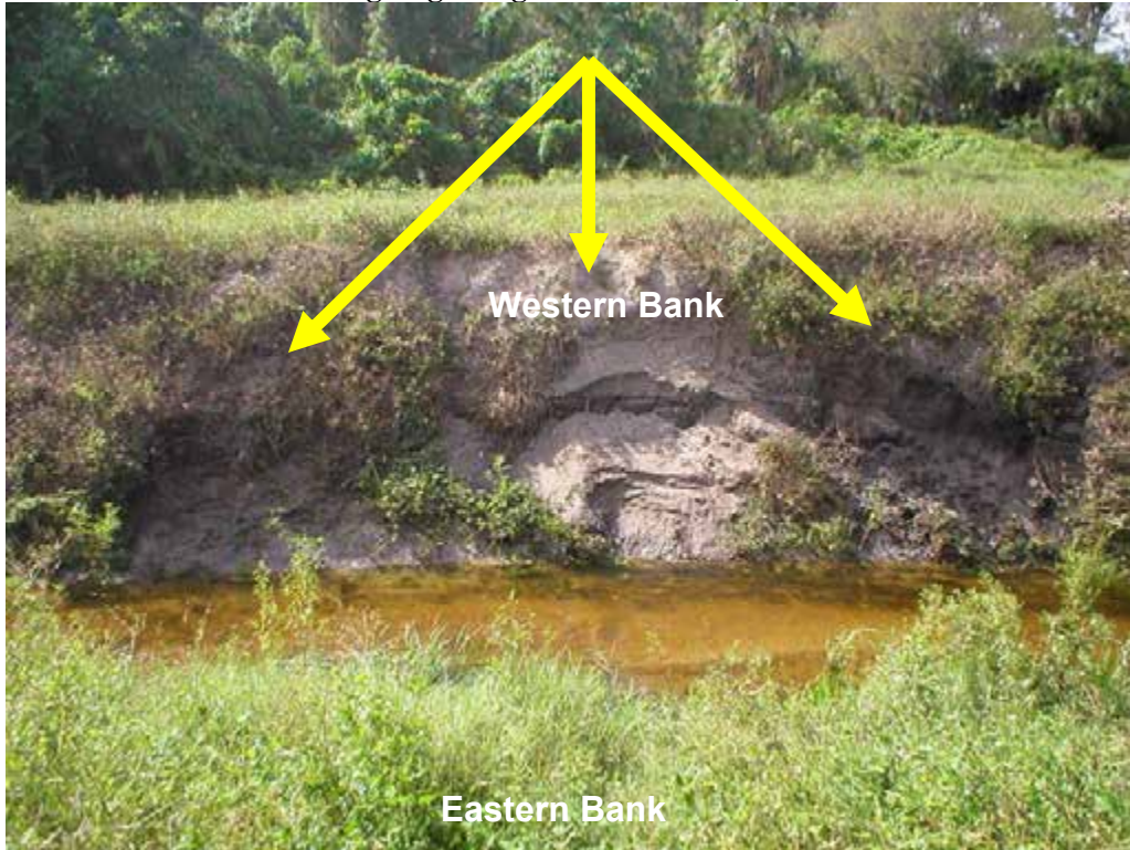
Photo 12 - System 3 Erosion along Eastern and Western Banks, May 2005
