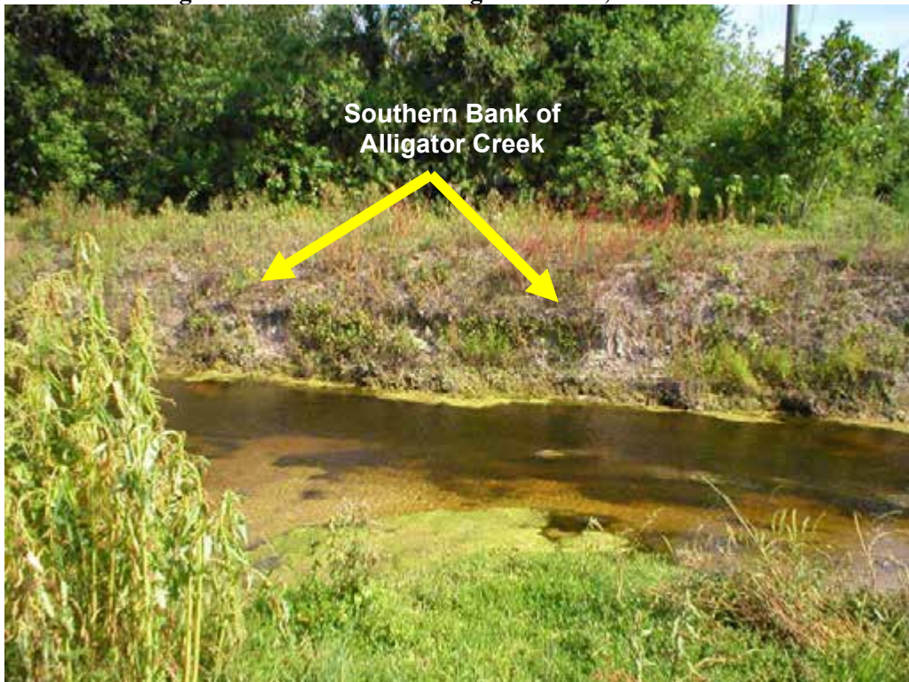
Photo 4 - System 1 - Segment 1 Undercutting of Southern Bank at Alligator Creek, November 2005
