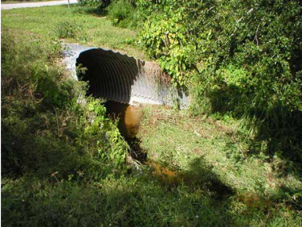
Photo 23 - System 5 - Segment 1 Culvert beneath Baffin Road, October 2005
