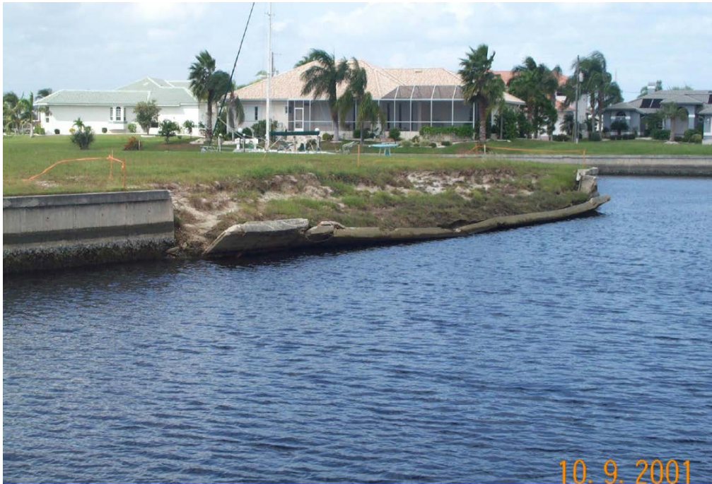
Failed Seawall
