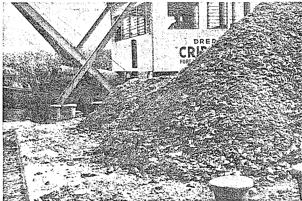
Spoil Piled On Barge Ready For Removal
