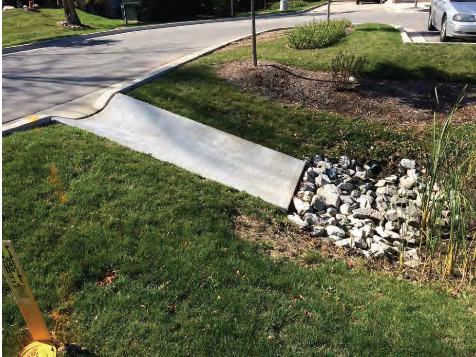
Figure 59 - Concrete Flume Example
