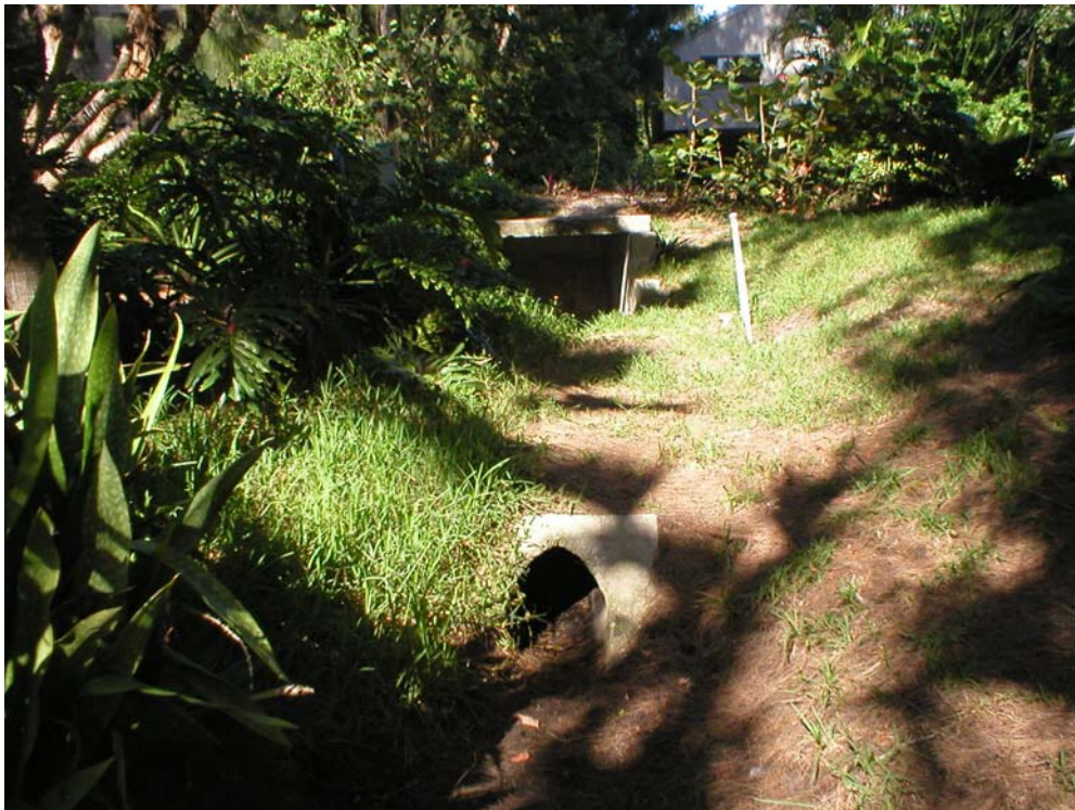
Figure 5. Outlet pipe BA1 discharging above water level.
