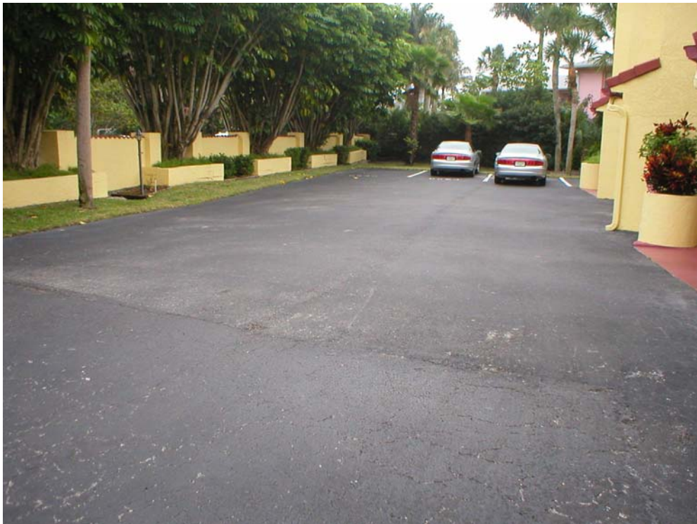
Figure 13. Parking lot west of Midnight Pass Rd. upstream of outfall SP2.
