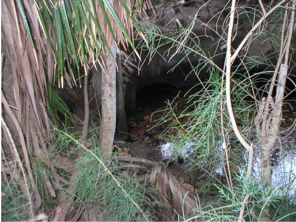
Figure 14. Outfall SP2 discharging below water level
