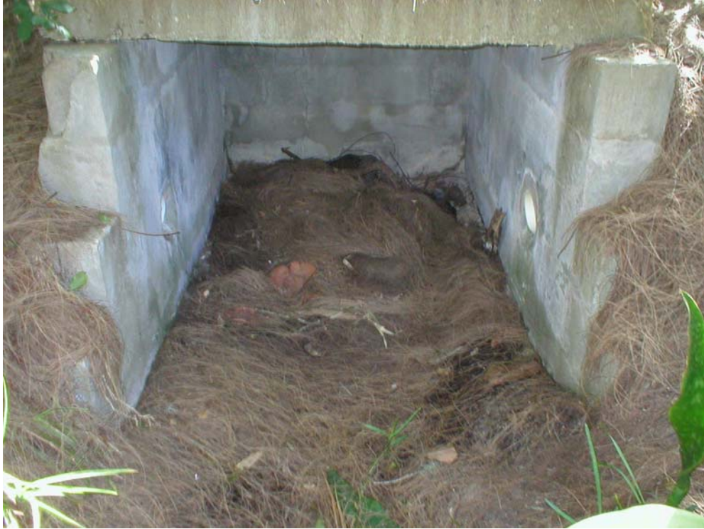
Figure 4. Northern end of culvert on Sea Plume Way upstream of outfall SP1.
