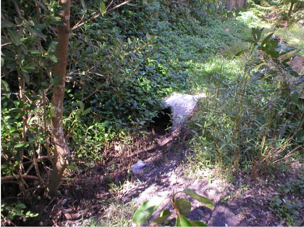
Figure 6. Outlet pipe SP1 discharging above water level.
