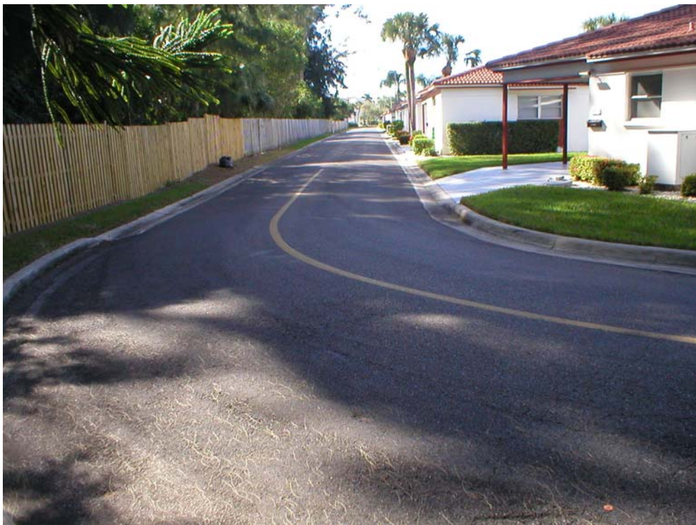
Figure 11. Looking west on Vista Hermosa Cir. from inlet upstream of outfall SP1.
