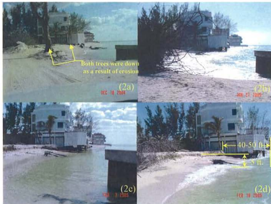
Fig.2 An acceleration of beach erosion occurred at the end of the Blind Pass bulkhead, north of 9250 Blind Pass Road (Plodzien). From December 16, 2004 to February 18, 2005, an estimate of 40-50 feet wide and 3-5 feet height of beach erosion was observed in a two-months period, undermining the pile-supported house and threatening its entry way, septic system and the road.
