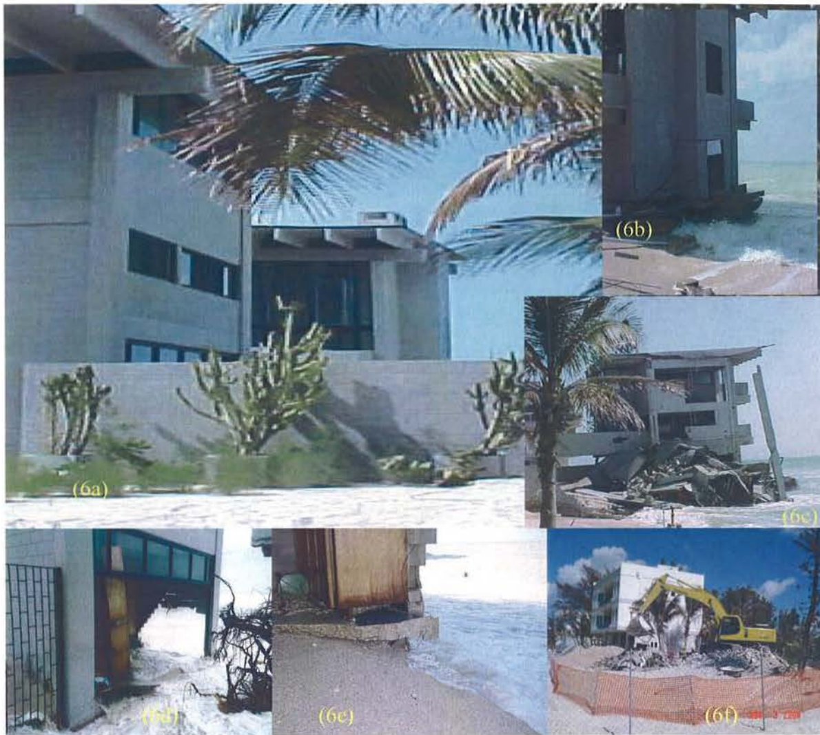
Fig.6 As a result of beach erosion, one of the two Mrs.Burns' residences collapsed into the Gulf of Mexico in March 2003. Her second residence sustained structural damage in Hurricane Ivan and was demolished by the County in late October 2004. (6a) Burns' two residences before collapsed. (6b) Undermining of the foundation by wave action. (6c) The west portion of the residence collapsed, and the County removed the debris in March 2003. (6d) Storm waves washed out a portion of the front wall in Hurricane Ivan. (6e) Waves undermined the foundation. (6f) Pursuant to Sarasota County Building Code Section 22-34(3), the County demolished the second Burns' residence.
