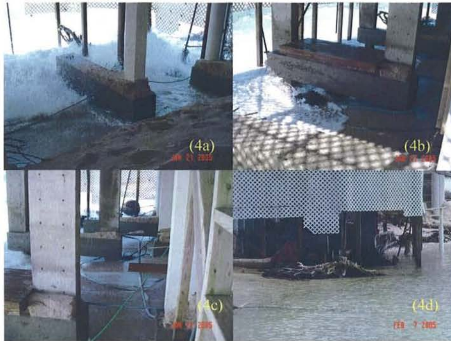
Fig.4 Due to shoreline erosion, wave action undermined Mr. Plodzien's (#3 in Fig.1) pile-supported residence this winter. 4a, 4b&4c showed the pile caps were undermined by wave actions. (4d) The breakaway fence was damaged.
