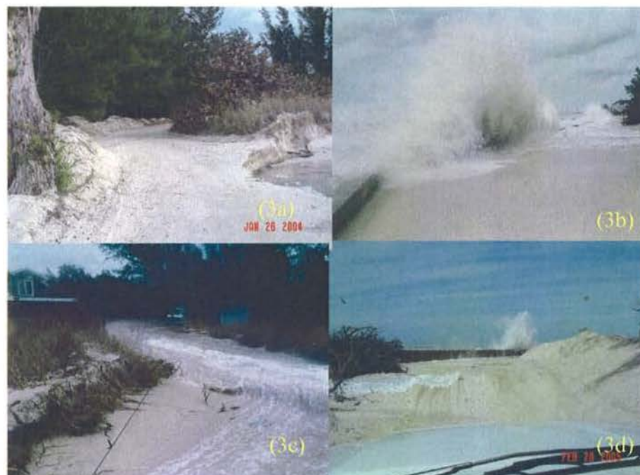
Fig.3 Damage to the Blind Pass Road. (3a) Local scouring at the end of the bulkhead made the road un-passable last winter. (3b) Storm waves like this one destroyed a 275-foot concrete cap of the 510 feet long steel bulkhead (photo was taken on September 16, 2004 after Hurricane Ivan). (3c) Storm wave over-topped the bulkhead and washed portions of the road (photo was taken on September 16, 2004). (3d) The tree was washed out and the road is under direct threat.
