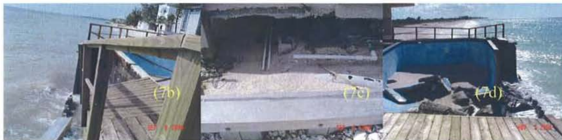
Fig.7 Property damages at Colkitt's gulf front residence (#6 in Fig.1). (7a) Colkitt's residence at 9230 Blind Pass Road. (7b) An aluminum bulkhead, pool and wood deck were damaged during Tropical Storm Frances on September 3 rd , 2004. (7c) House foundation was undermined by wave action. (7d) Aftermath after storm season.
