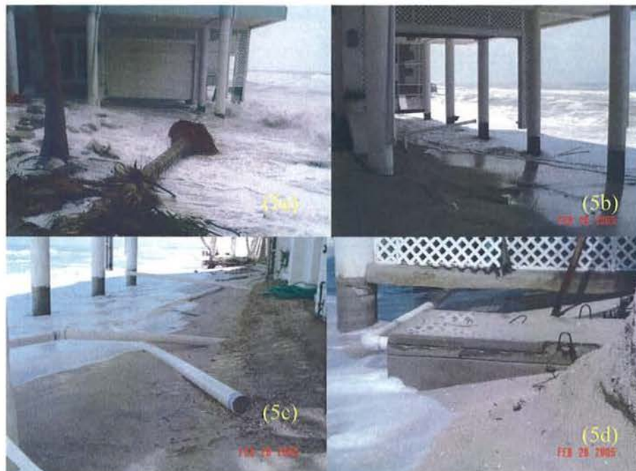
Fig.5 Dr. Fassy's pile-supported residence was undermined by wave actions. (5a) & (5b) Former garage area was completely washed away, the entryway was directly under threat. (5c) Sewage pipes were washed out. (5d) Septic tank was exposed and under threat.
