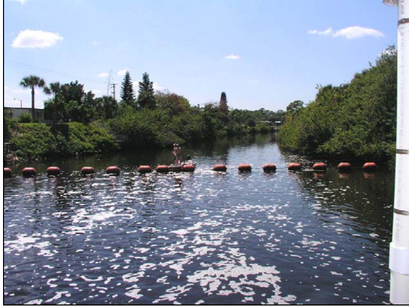
Area 9 - Channel from Area 9 would connect to Shakett Creek immediately south of this location.
