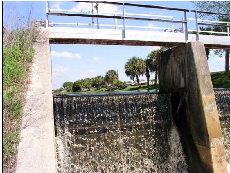
Area 9 - Cow Pen Slough control structure north of Area 9 channel.
