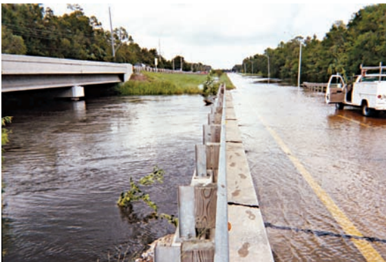
Figure 4. Views of Trout Creek near Sulphur Springs (site 24) on downstream side of bridge. Top—view when creek was at gage height of 37.01 ft and flow of 25 ft 3 /s on October 2, 2003. Middle—view during flood on September 7, 2004, at stage 6 ft higher and flow of 1,610 ft 3 /s. Bottom—view of west bound traffic lane (State Highway 581) overflow discharge on September 7, 2004. Photographs taken by R. Carson and G. Baraket, U.S. Geological Survey.
